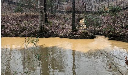
During the wet winter months, we spend time focusing on construction stormwater violations. Pictured above shows failures in best management practices and violations of sediment leaving the site after a rain event. We collected turbidity samples and are monitoring the situation.
